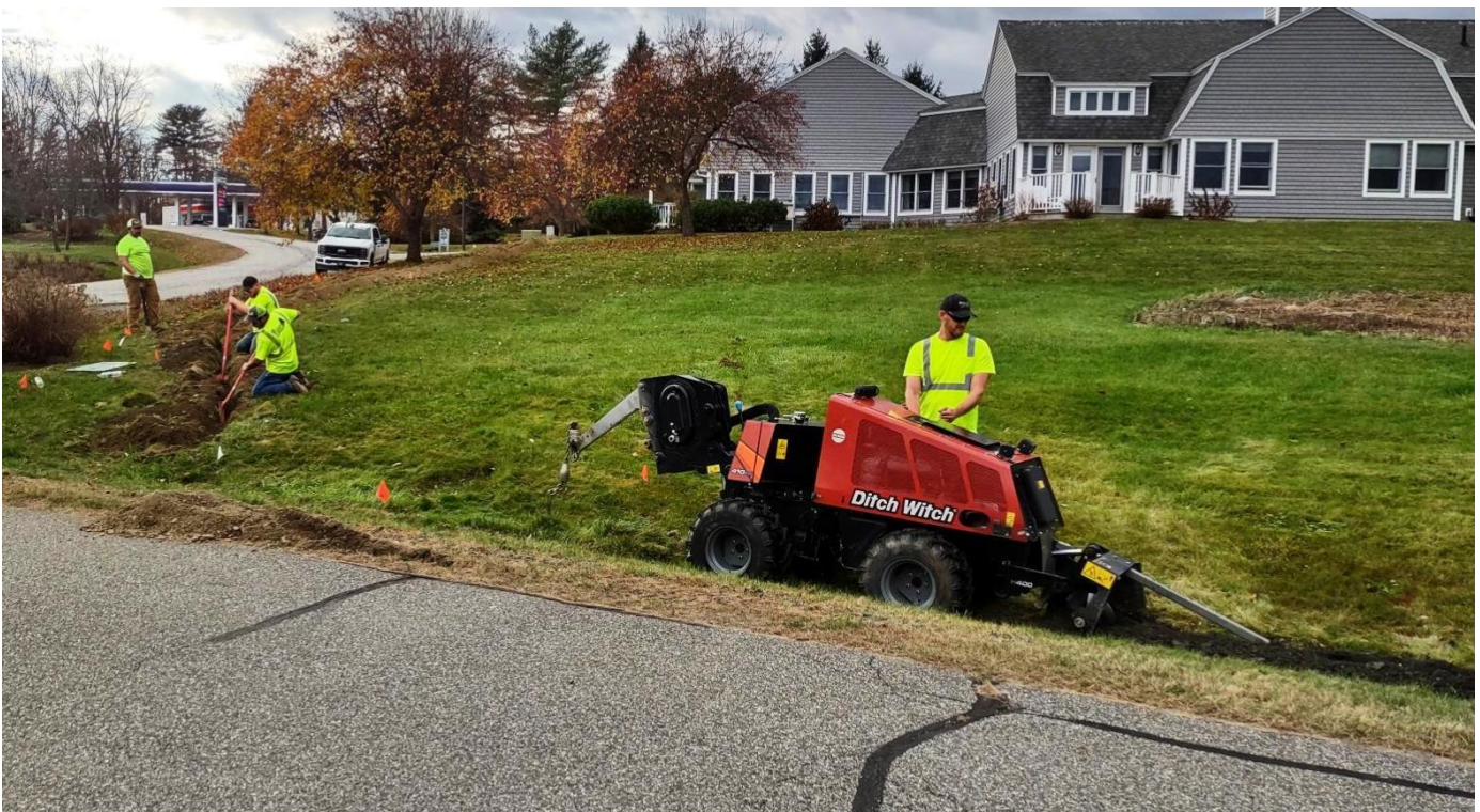
Fidium Fiber was on campus putting in fiber optic cable.
